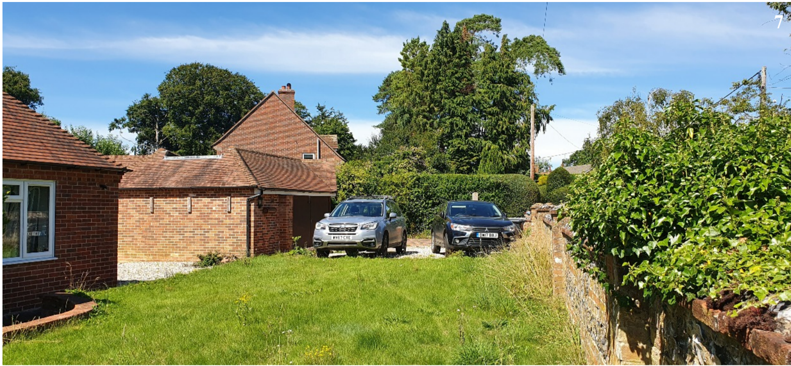
7. View gained from the front garden, showing relationship and distance between the bungalow, the outbuildings and adjacent property
